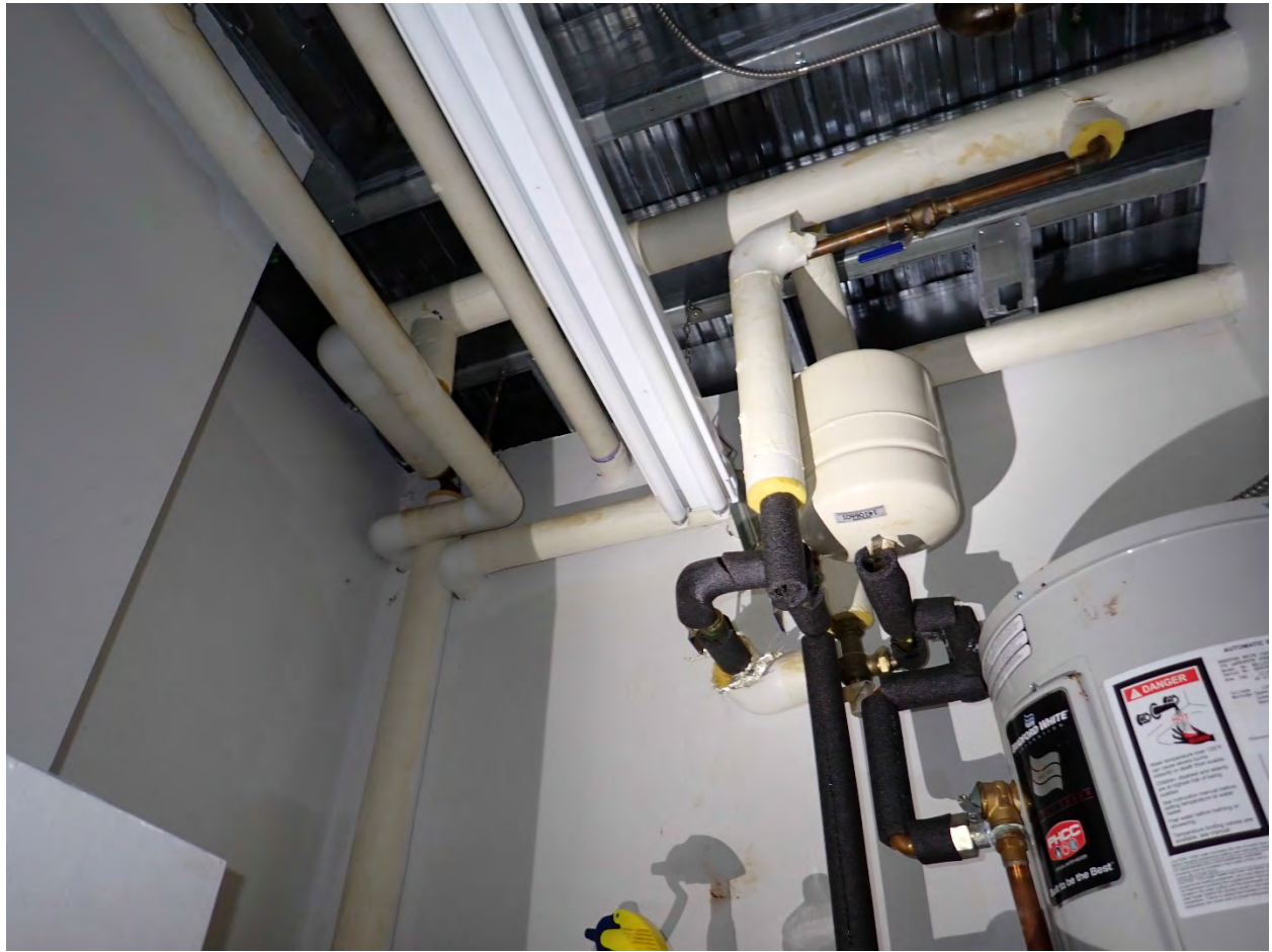
Non-Suspect Fiberglass Pipe Insulation and Zeston Fittings
